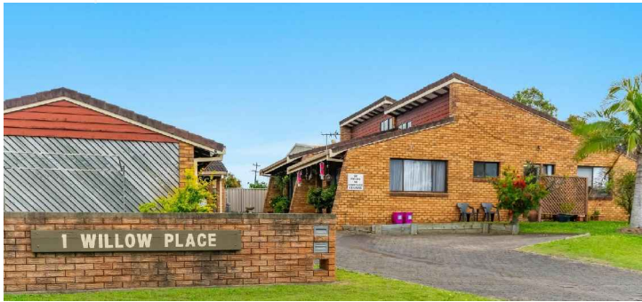
EXISTING 1 STOREY TOWNHOUSE DEVELOPMENT 1 WILLOW PLACE
