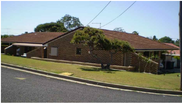
EXISTING 1 STOREY VILLA DEVELOPMENT 26 TALLOWOOD AVE
